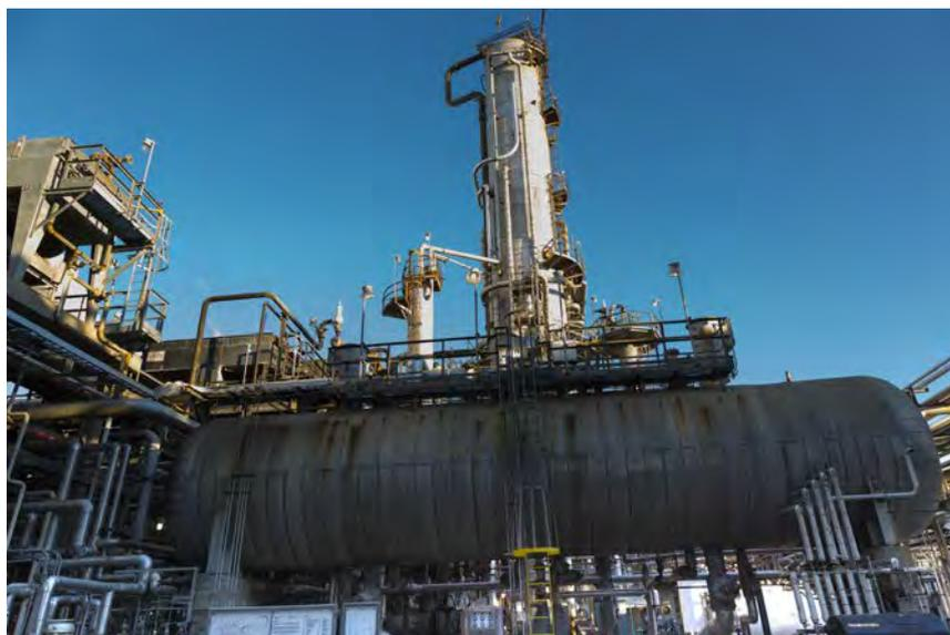
**Figure 2.** Desalter and crude tower at a US refinery.
